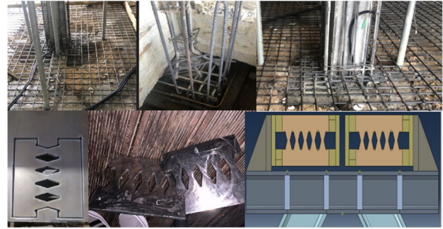
Fig.1 In Execution!! Rehabilitation Tirana Hospital (Autor:F.Gashi , prof.Markel Baballeku) ecc.
