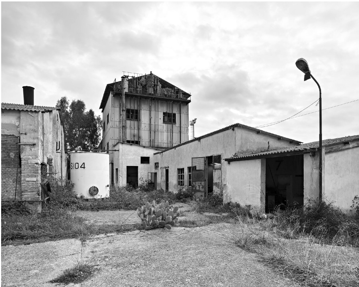
Fig. 7 Abandoned factory, Solarussa, Italy. Photo: D. Viridis
