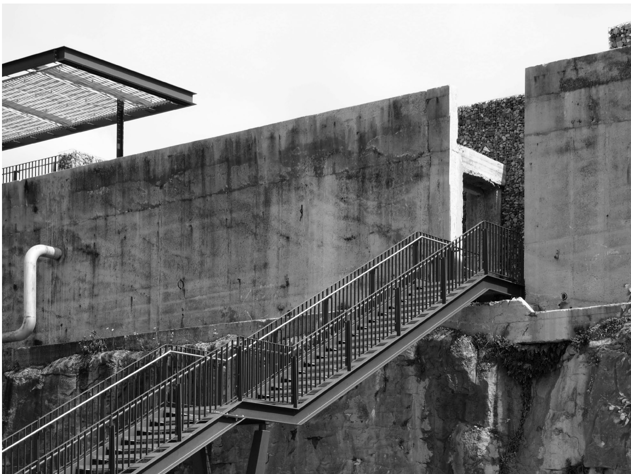
Fig. 9 McGregor Coxall, Ballast Point Park, Sydney, Australia. Photo: D. Hill
