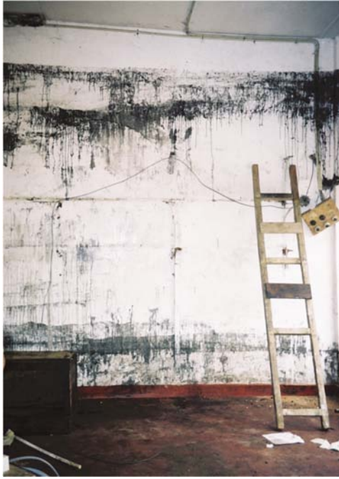
Fig. 4. Characteristic indoor sea sand mark left behind by the tsunami in the coastal zone of downtown Hambantota, south Sri Lanka. This is one of the locations where the maximum water level of h \sim 11 m was measured.
