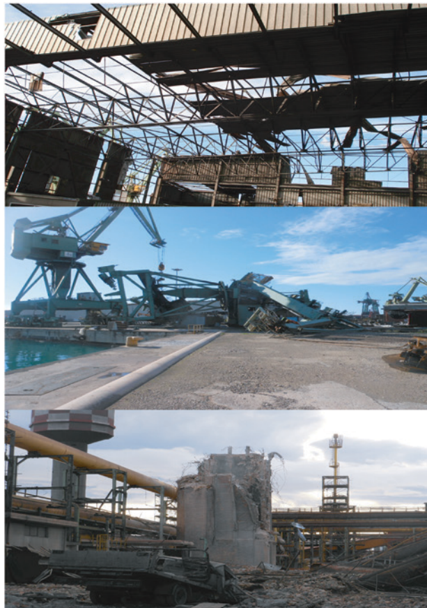
FIG. 3. (top) Collapse of metal structures in the port area; (middle) a crane weighing several tons lifted; and (bottom) a concrete chimney completely destroyed (courtesy ILVA S.p.A.).
