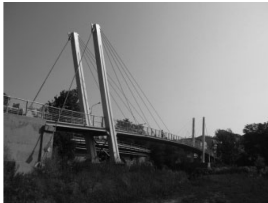
Figure 1. A view of the tested cable-stayed pedestrian bridge.
