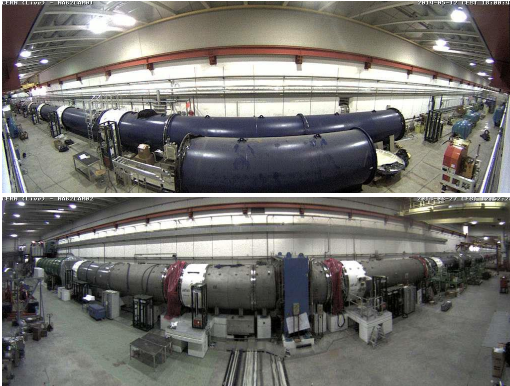
Figure 2. Live webcam pictures taken before and after the completion of the installation of the decay beam pipe of the NA62 experiment at CERN.
