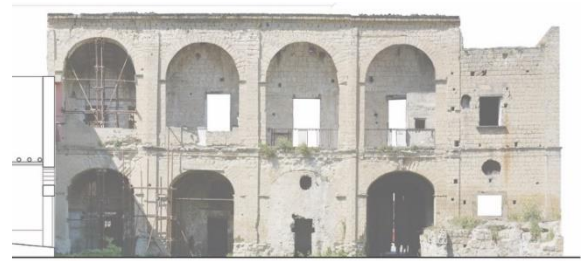
Figure 10. Conservation status of Masseria San Lorenzo : section of the court. ©Restoration project of Masseria S. Lorenzo (NA), G. Coppola, M. De Rosa, F. Guarracino, M. Iengo, F. Ridente, Course or Laboratorio di Restauro architettonico, R. Picone a.a. 2018/19
