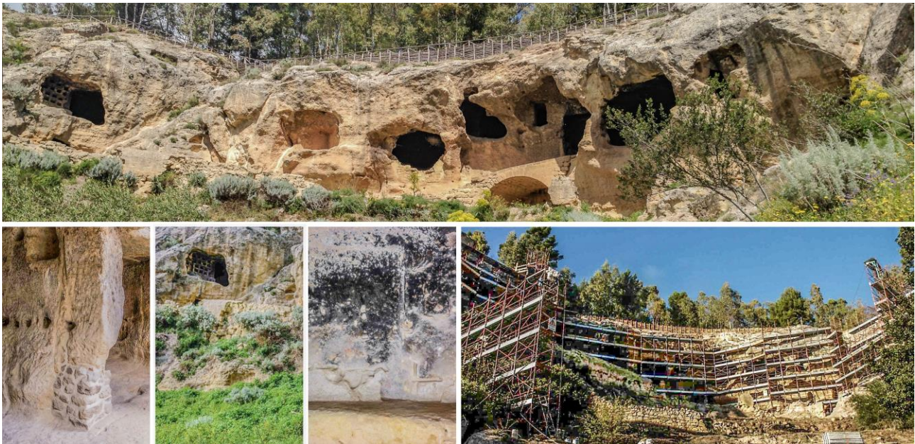
Figure 2. The Canalotto Valley: today and during the consolidation works undertaken in 2000.
