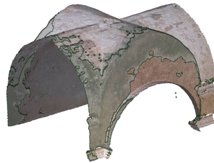
Figure 8. Case 1: superimposition of cluster 1 (biological colonization) to the original point cloud to the original point cloud
