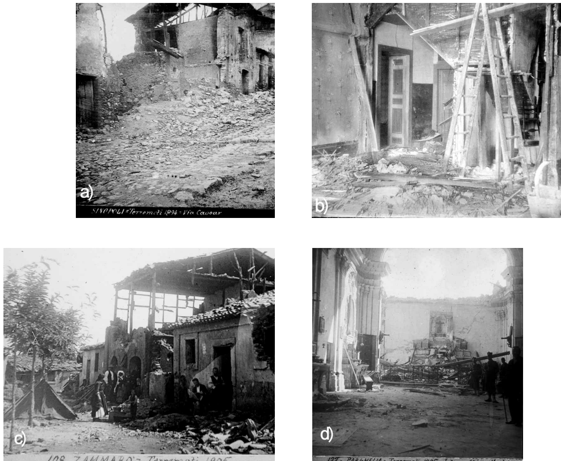
Figure 3. Some examples of earthquake images taken from the stereoscopic viewer slide set: a) Collapsed buildings in the Calabrian village of Sinopoli (1894 earthquake); b) interior of a semi-destroyed house in the Sicilian city of Messina (1894 earthquake); c) survivors in front of their semi-destroyed homes in the Calabrian village of Zammarò (1905 earthquake); d) total collapse of the roof in the Mother Church of Parghelia, Calabria (1905 earthquake).
