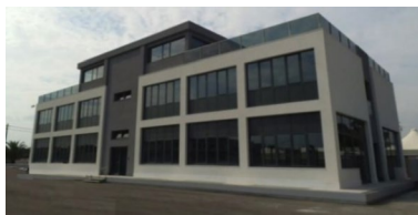
(a) East view of the building.
