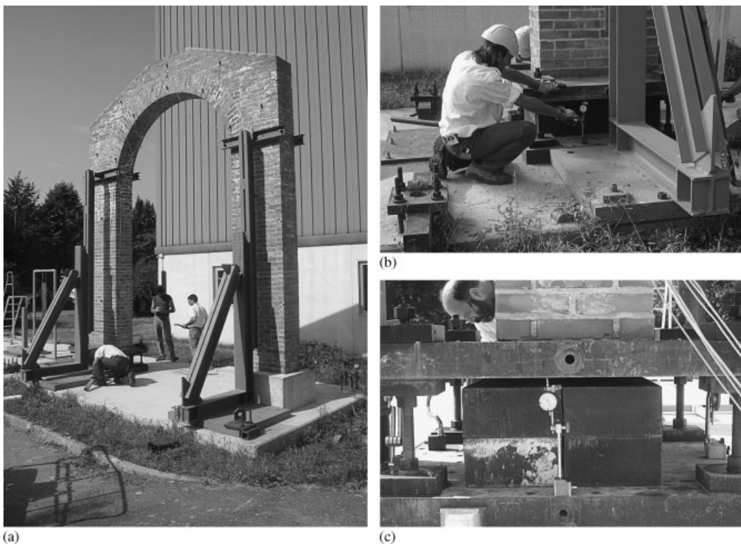
Figure 17. Settlement: (a) provisional structure and (b) and (c) lowering operations.
