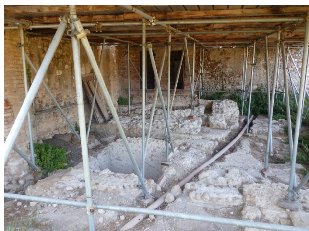
Figure 2: view of the archaeological area. The temporary roof cover lies directly on the archaeological structures, only protected by some protective layer.
