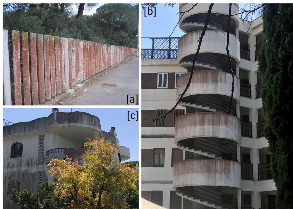
Fig. 3 Widespread and distribution of BP. a The abundance of the red-orange biofilm in the favourable condition of Grassi hospital. b The differences of colonisation related to the aspects (Santa Severa). c The ecological transition from red-orange BP to black BP (S. Marinella)
