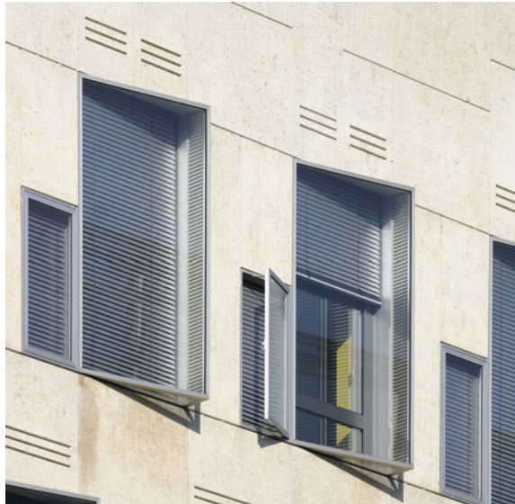
Fig. 1.4 Façade with integrated classic windows for direct air exchange (DKV Insurance Company HQ, Cologne, arch. Jan Störmer Architekten, 2005)
