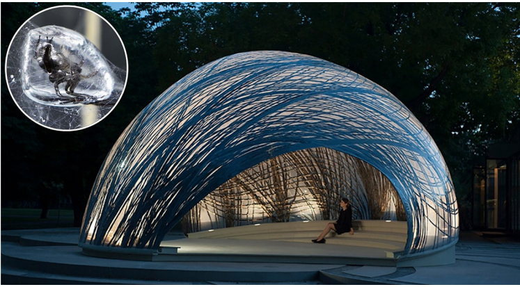
Fig. 1 ICD/ITKE Research Pavilion 2014-15. Demonstrative pneumatic fiber-reinforced pavilion inspired by the water spider underwater nest construction and made using robotic fabrication processes. Authors: Institute for Computational Design and Construction (Prof. A. Menges) Institute of Building Structures and Structural Design (Prof. Dr.-Ing. J. Knippers). Source/Credits: ICD/ITKE University of Stuttgart. https://www.itke.uni-stuttgart.de/research/icd-itke-research-pavilions/icd-itke-research-pavilion-2014-15/
