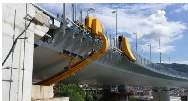
Figure 1. Robot installed on the new Viaduct on the Polcevera river.
