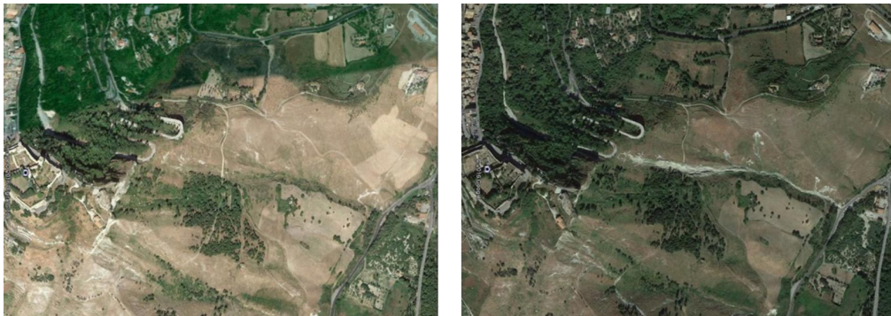
Fig. 1. (a) the area prior of the debris flow; (b) the area after the debris flow.
