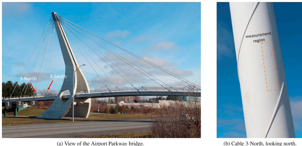
Fig. 2. Field measurements on the Airport Parkway bridge in Ottawa, Canada.
