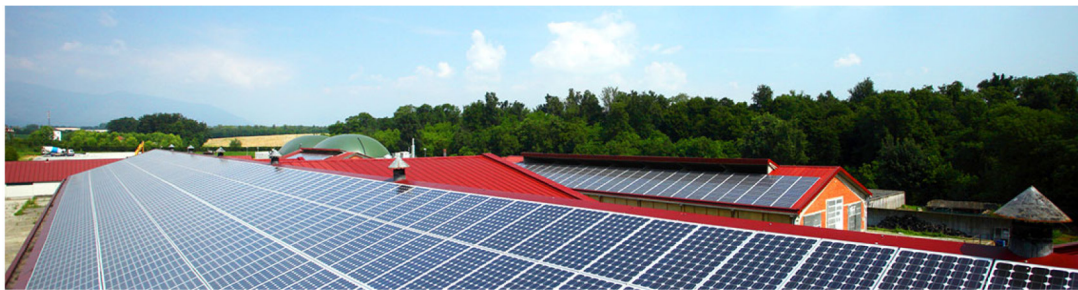
Fig. 1. Existing PV roofs of "La Bellotta".
