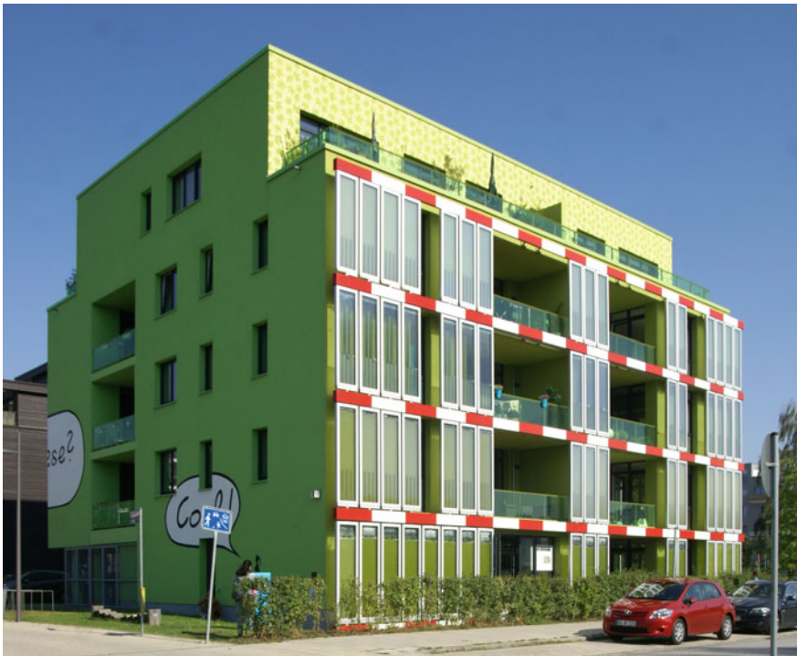
Fig. 3.25 BIQ (arch. SPLITTERWERK, Arup GmbH, B+G Engineers, Immosolar, 2013)
