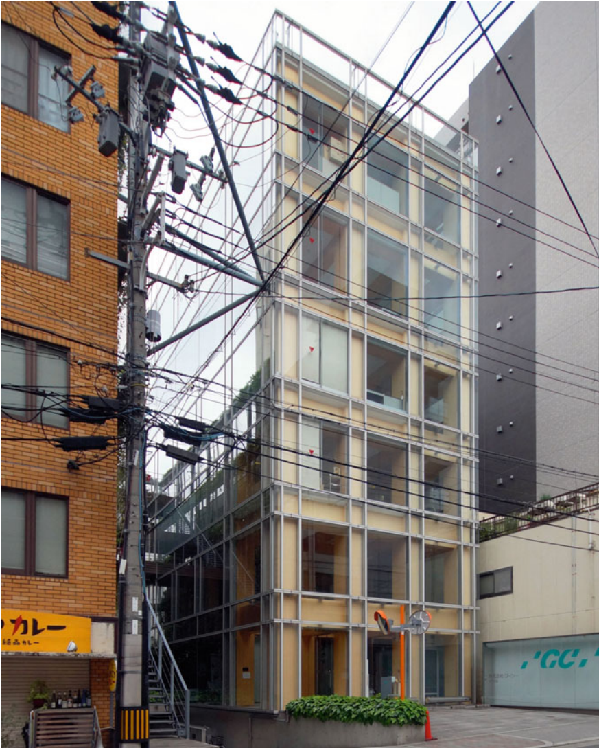
Fig. 3.13 Bio-based façade elements protected by external layer of glass, as implemented in GC Osaka Building (arch. Shigeru Ban Architects, 2000)
