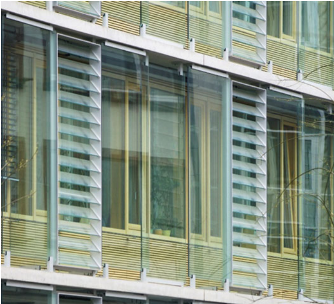
Fig. 3.14 Double-skin façade with bio-based aesthetical components protected by glass and ventilation layers—FH 1 building at the campus of Frankfurt University of Applied Sciences (arch. Heribert Gies Architekten, MainzVoigt & Herzig Architekten & Ingenieure, 2007)
