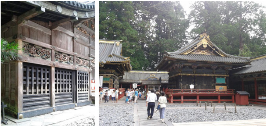
Fig. 3.11 Sculptured façades of ancient Japanese buildings
