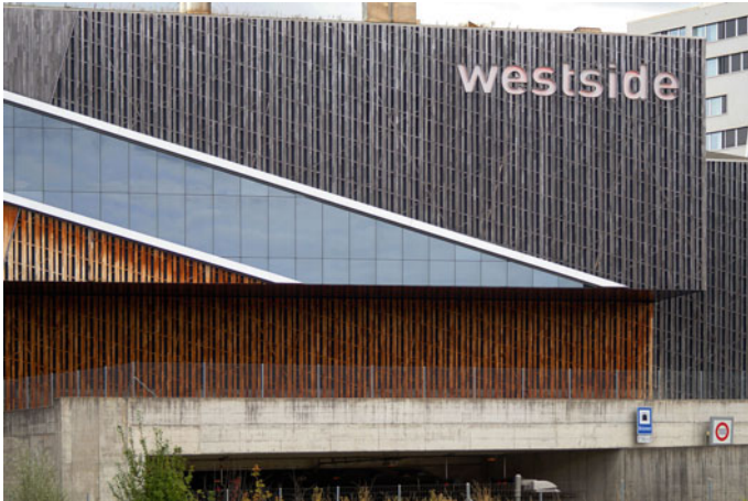
Fig. 3.18 Vertical orientation of cladding in Westside Shopping and Leisure Centre in Bern-Brunnen (arch. Daniel Libeskind, 2008)
