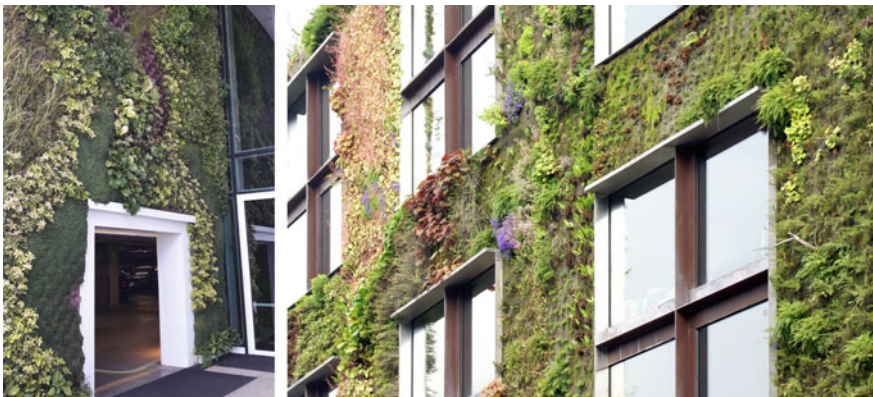
Fig. 3.26 Green façade on blind sections of the wall
