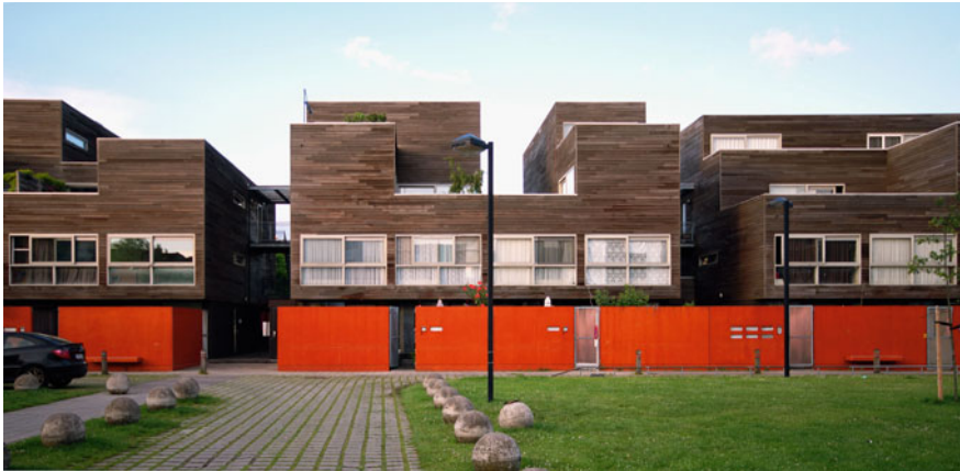
Fig. 3.17 Single-side exposed bio-based façade as implemented in Hollainhof housing development in Ghent (arch. Neutelings Riedijk, 1998)
