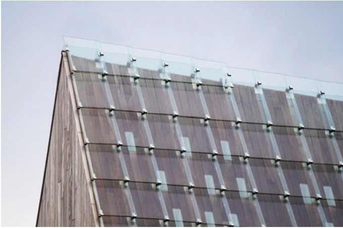
Fig. 3.15 Bio-based façade elements protected by external layer of glass, as implemented in Market Hall in Ghent (arch. Marie-José Van Hee + Robbrecht & Daem, 2012)
