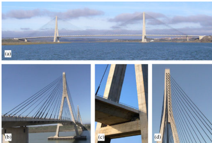
Figure 1. The International Guediana Bridge: (a) lateral view; (b) perspective view from Spain; (c) details of the deck–tower connection; and (d) details of the stay cables.
