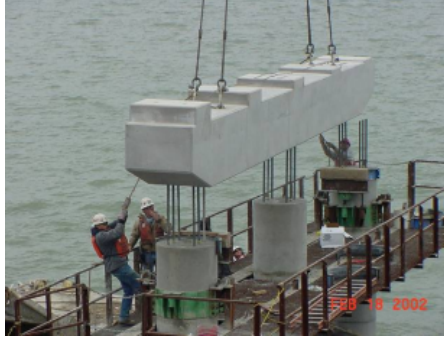
(a) Erection of precast pier cap [11]
