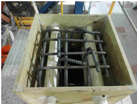
(e) Reinforcement of loading block
