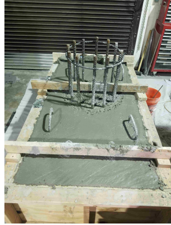
(b) Casting of concrete
