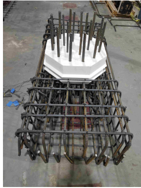
(a) Reinforcement cage
