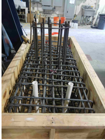
(a) Reinforcement cage
