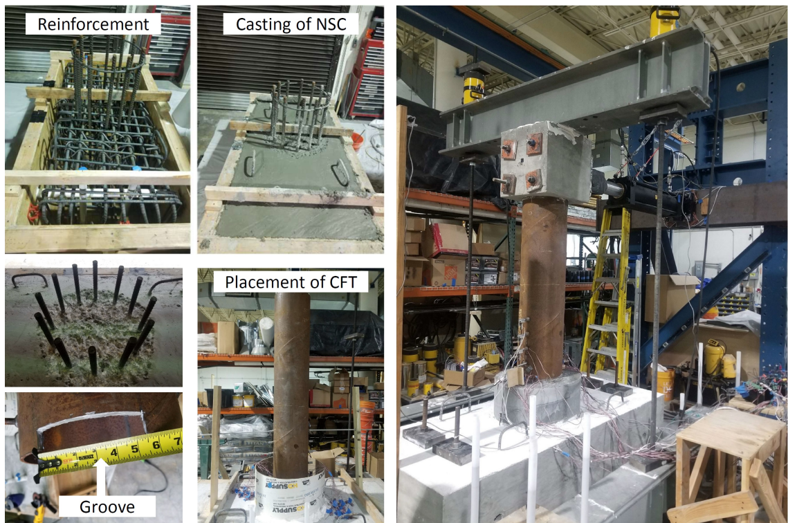
Figure 3.6: Construction of encased connection (specimen-2).
