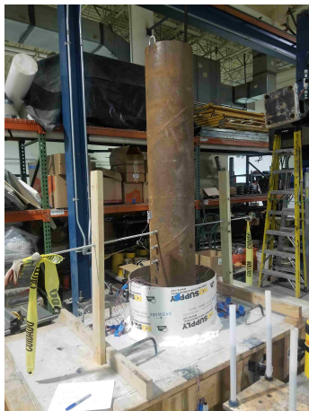
(e) Casting of UHPC
