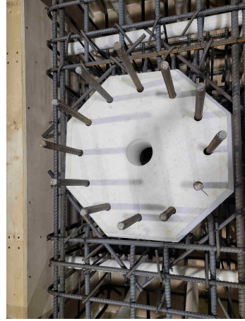
(b) Dowel arrangement
