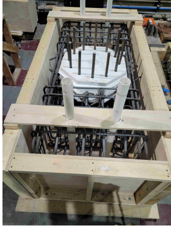
(a) Reinforcement cage
