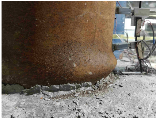
(c) Buckling of tube at 5\Delta y
