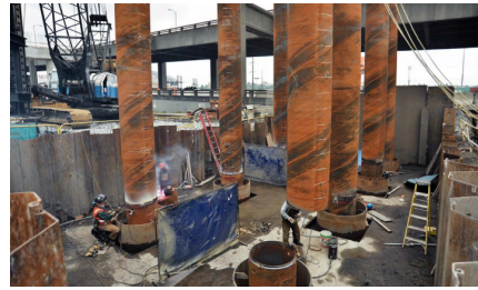
(b) CFT for substructure [14]
