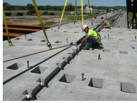
(b) Connection for precast deck panels [10]
