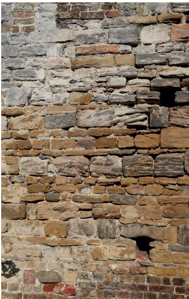
FIG. 1 Damme, OLV-kerk, zuidwand van de westtoren. Parement met lappendeken van verschillende natuursteensoorten. Damme, Church of Our Lady. Southern side of the western tower, with its patchwork of different types of ashlar.
