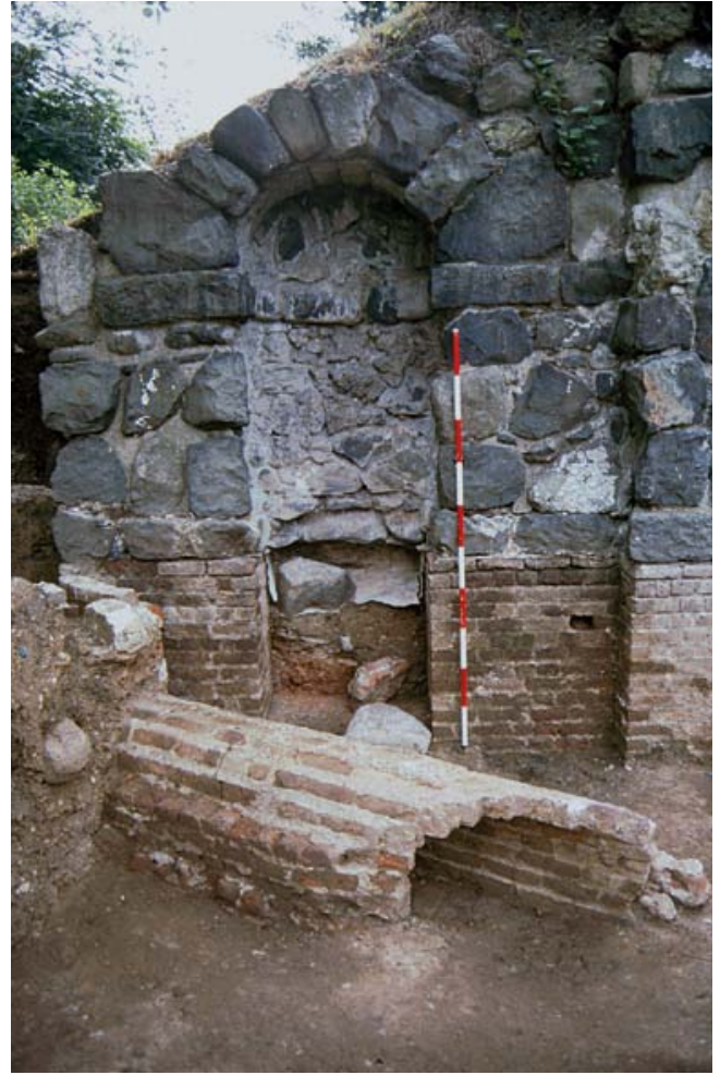
FIG. 36 Foundations and other substructures revealed by excavation beneath the Cascade which was built to a design by William Kent in about 1738 at Chiswick House in West London. Scale length, 2 m.
