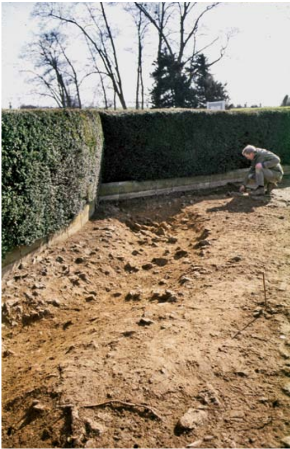
FIG. 30 Re-excavation of the Great Garden at Kirby Hall in Northamptonshire, England showed the inaccuracy of previous reconstruction in the 1930s.
