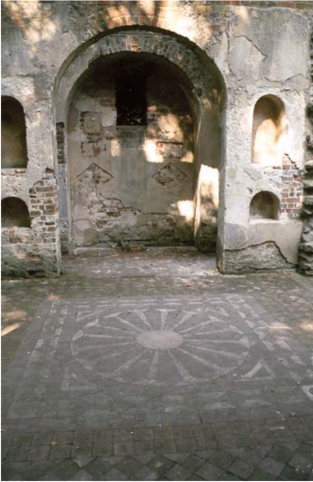
FIG. 35 The floor of the Mausoleum at Painshill Park in north Surrey, England has been relaid using the results from previous archaeological investigation.
