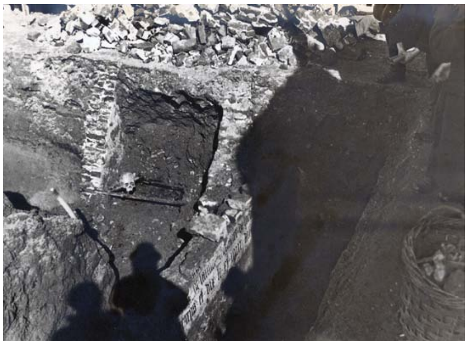
FIG. 66 Aangesneden grafkelders bij de aanleg van de commandopost in 1941. Discovery of brick vaults during the construction of the shelter in 1941.
