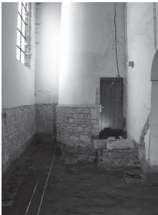
14 Traptoren in de zuidwestberging. Spiral tower in the southwest chapel.
