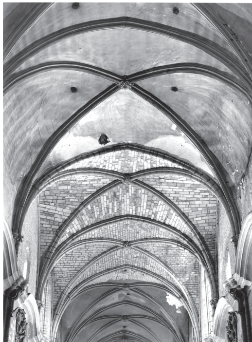
19 13de-eeuwse stenen kruisribgewelven en 18de-eeuwse schijngewelf in pleister. 13th-century stone cross-rib vaults and 18th-century fake vaults in plaster. (© Brussel, IRPA-KIK, B158475, ca. 1940)
