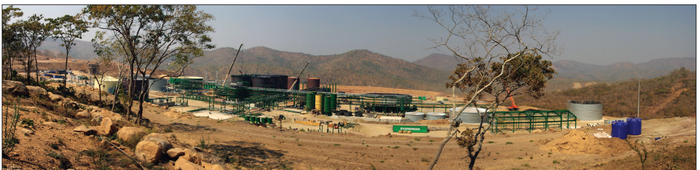
Plant construction at Kayelekera (photo courtesy of Paladin Energy Ltd).
