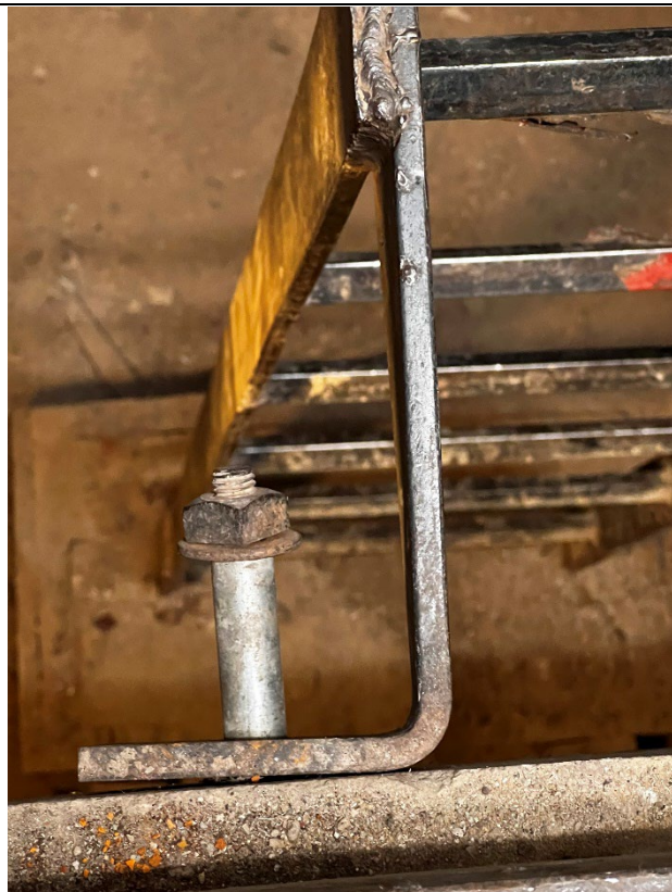
Photograph: 16 Close-up of access ladder, left side.
