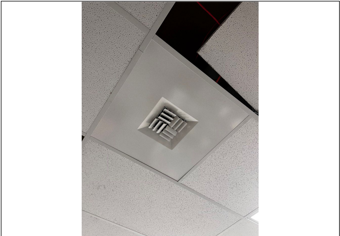
Photograph: 10 Ceiling vent.
