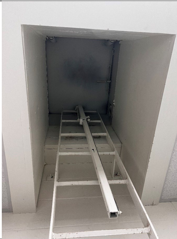
Photograph: 11 Ladder to roof access.
