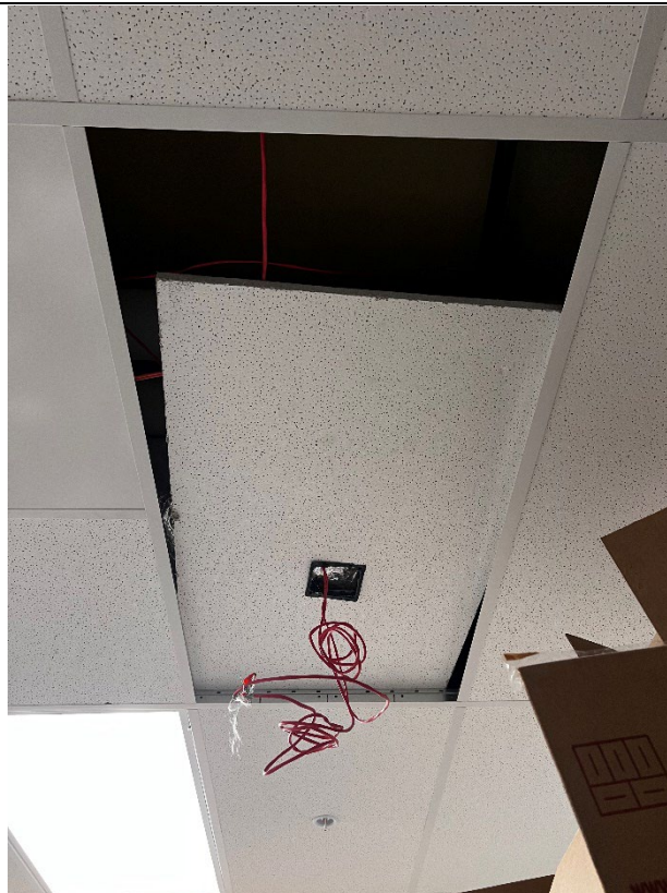
Photograph: 12 New wiring being run into room via ceiling.
