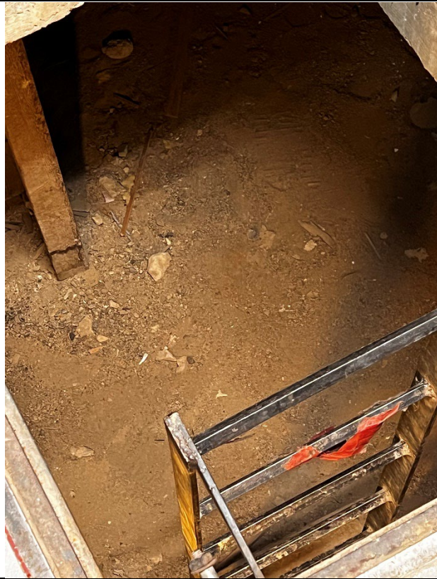
Photograph: 17 Earthen floor of crawl space.
