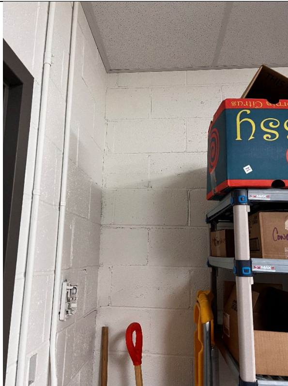
Photograph: 5 Front left corner of storage room, facing south.
