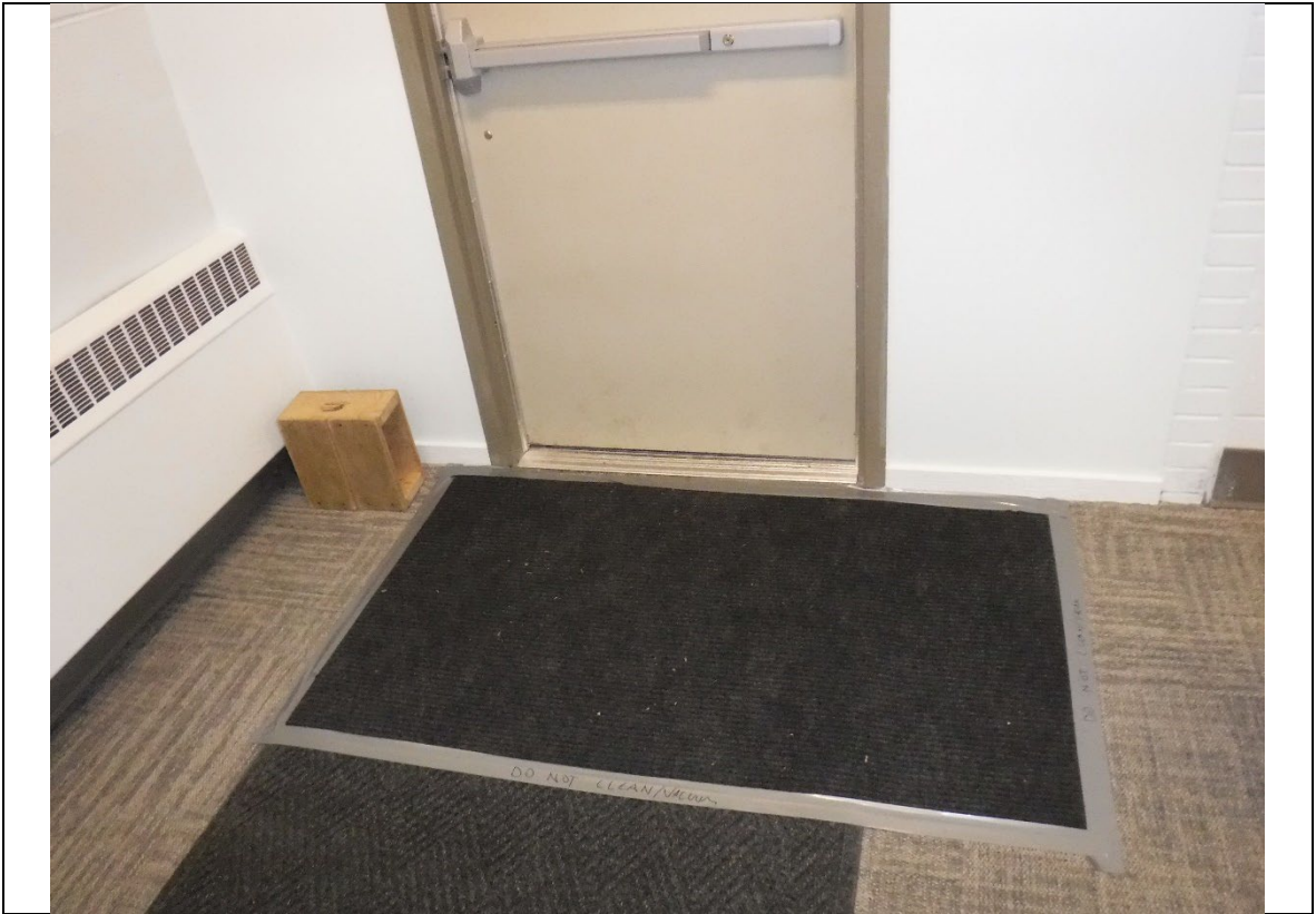
Photograph: 1684 | Floor surface sample, back entrance from playground (S-0013-D-FM-03-20230523)
