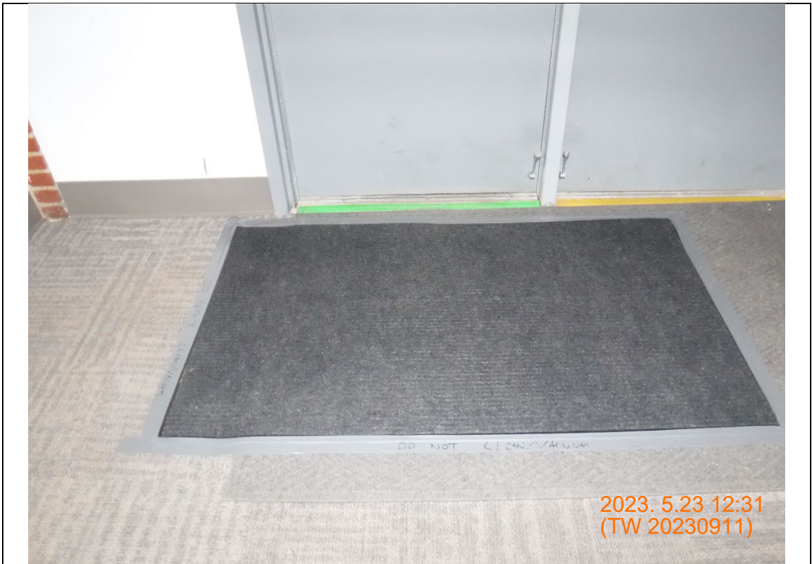
Photograph: 1682 Floor surface sample, main west entrance by front office (S-0013-D-FM-01-20230523).
