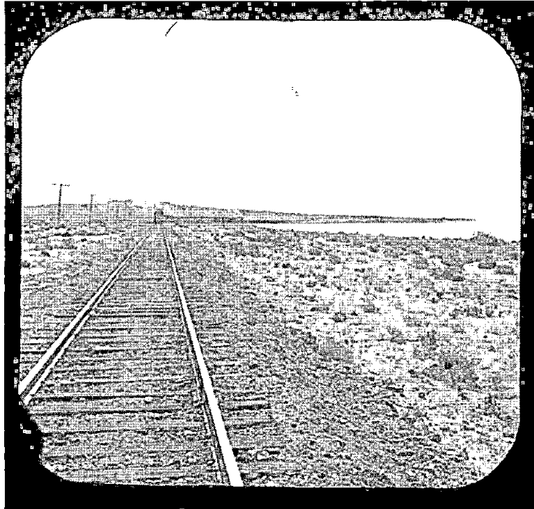
The Southern Pacific tracks were flooded by rising waters. They were moved to a higher location east of the Salton Sea.
