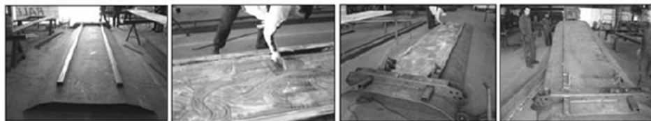
Figure 14 Assembling process of the panel over the floor plate
