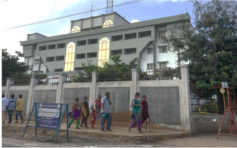
Figure 7.30 : An unfinished foot path along an arterial road in Coimbatore
