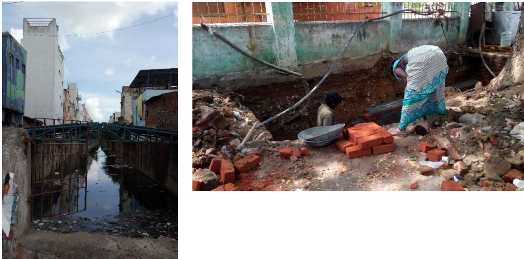
Figure 7. 9: (L) Dilapidated state of a waterway in T. Nagar (R) Construction of a stormwater drain (mason assisted by his wife)
