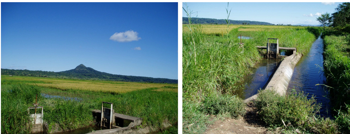
Figure 20: 5.6 Water diversions (water use) for irrigation in Limphasa Rice Scheme
