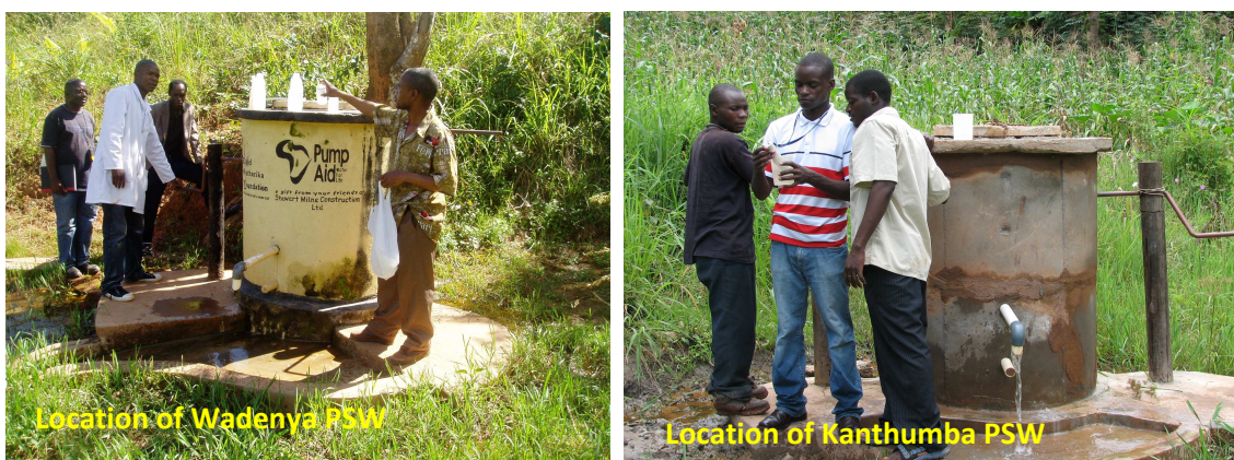
Figure 41: 7.3 Protected shallow wells located in low-lying wet areas (35-53% slope)
