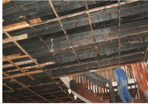
Figure 62 Fire damaged floor and roofing timbers uncovered during restoration of the 1903 Sacks Futeran warehouse building. District Six Museum archive.
