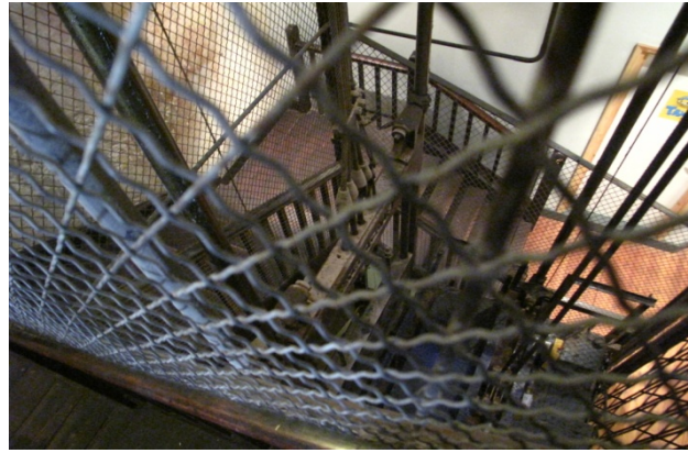
Figure 68 Enclosed lift shaft with safety fencing and wooden staircase. Homecoming Centre. HH-R.
