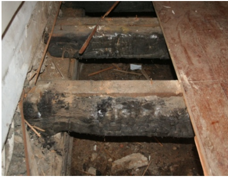
Figure 62 Fire damaged floor and roofing timbers uncovered during restoration of the 1903 Sacks Futeran warehouse building. District Six Museum archive.
