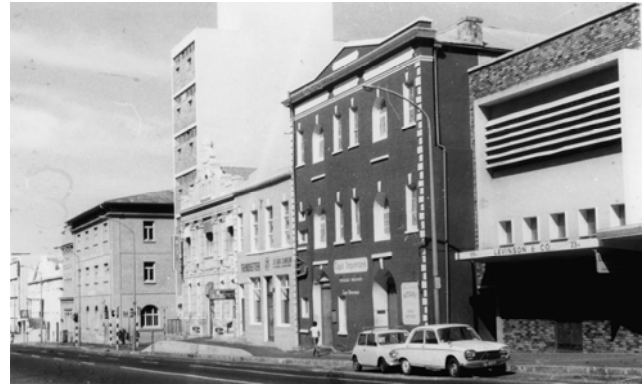
Figure 58 Sacks Futeran buildings, Buitenkant Street 1960s. NLSA.
