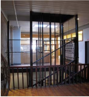
Figure 67 Otis lift shaft: Second floor Homecoming Centre. HH-R.
