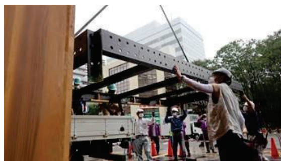
(e) Construction of the steel beam frame
