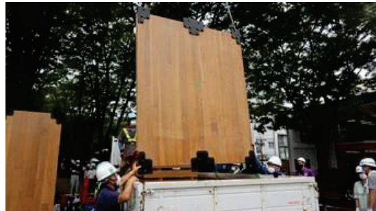
(c) Installation of the CLT walls
