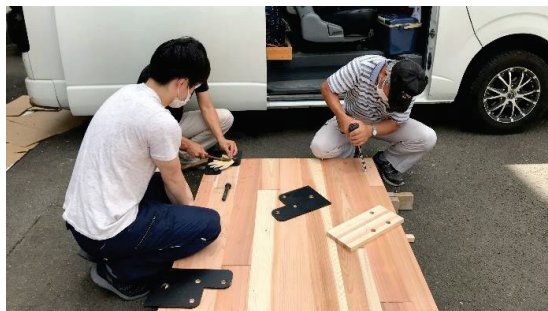
(a) Opening bolt holes for a CLT wall by a carpenter
