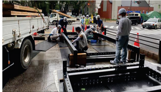
(b) Assembly of the steel base and beams on the ground
