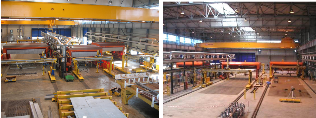
Fig. 23: Views of the PrePreFabrication Workshop
