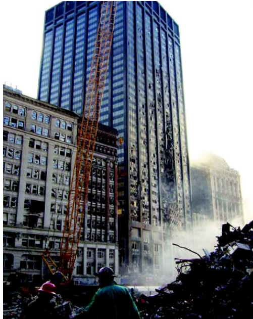
Figure 2.6. North face of Bankers Trust Building with impact damage between floors 8 and 23 (Smilowitz – FEMA, 2004)
