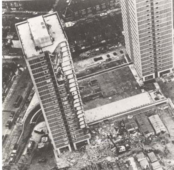
Figure 2.1. Ronan Point building after the accident [NISTIR 7396, 2005]
