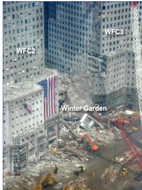
Figure 2.5. Photograph showing mild debris damage to WFC 2 and WFC 3, with the heaviest debris falling perpendicular to the west face of WTC 1 onto the Winter Garden [FEMA, 2002].
