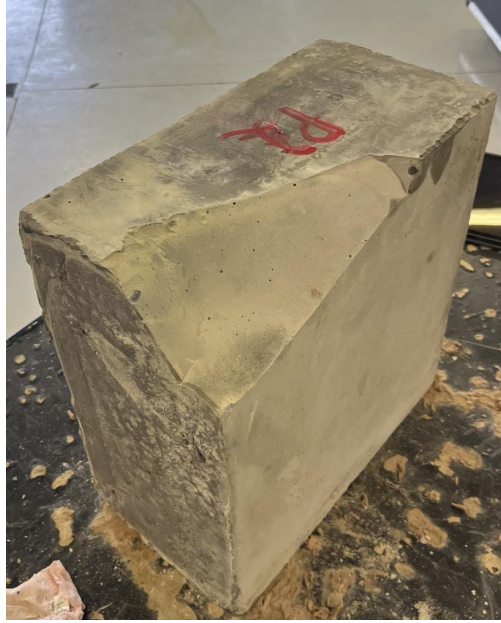
Figure 5.14: Grout Sample two with spherical defect
