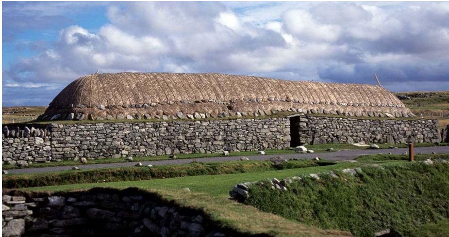
Figure 9: Arnol blackhouse, 19th century, Isle of Lewis. Preserved traditional blackhouse. Vernacular architecture in the Hebrides is a descendant of Norse architectural forms. The foundation of this house would be nearly identical to the foundation of a Norse period longhouse. Photo from Historic Environment Scotland.
