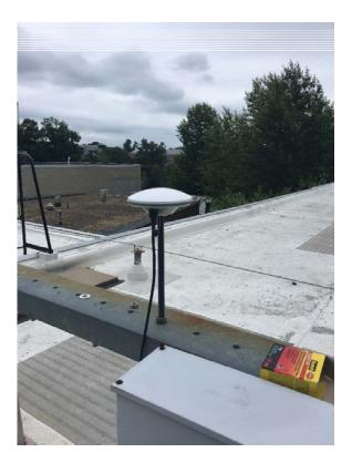
Figure 3: Harxon GPS500 antenna mounted on the rooftop of the CCOM wing of the Chase Ocean Engineering building.
