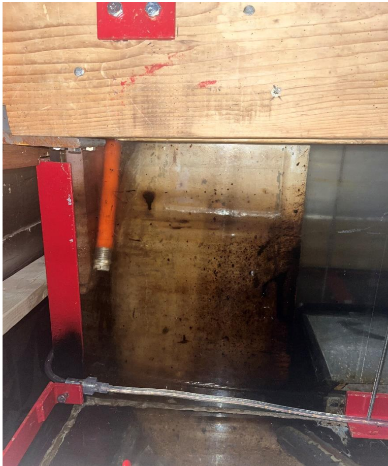
Figure 67: Location to secure hose in flume.
