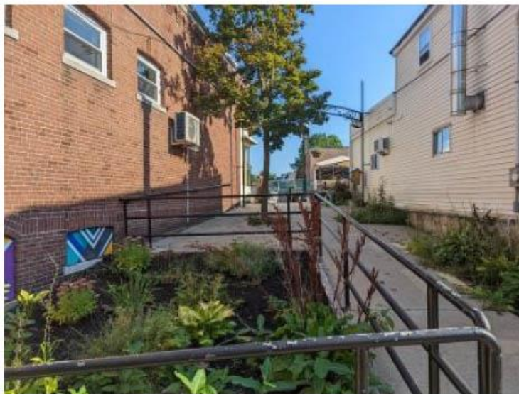
Walking path connecting Cocheco River to downtown Rochester. Construction fo a building is currently ongoing near the entrance of the path.
