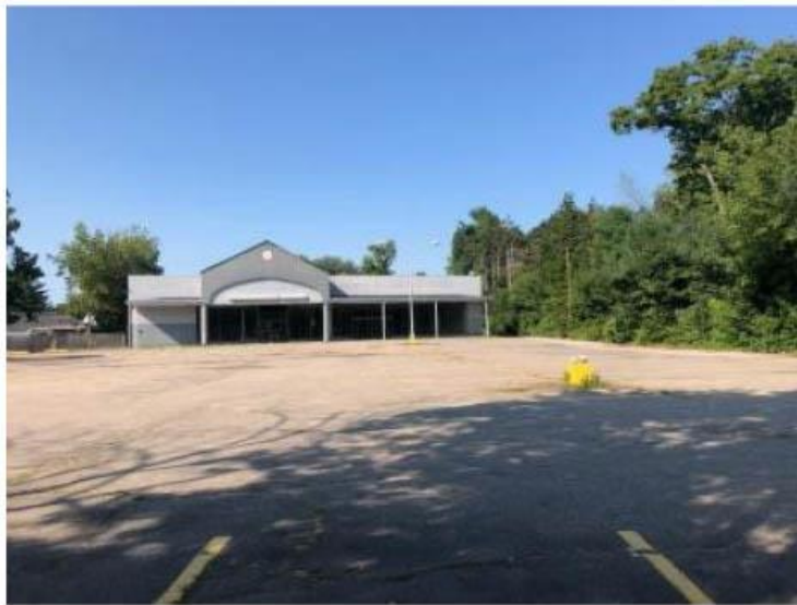
Currently empty building with development opportunities.
