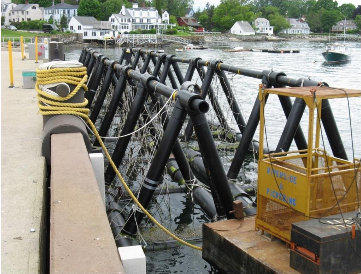
Fig. 4.7. Triton® barrier units separated and towed in to UNH Pier.
