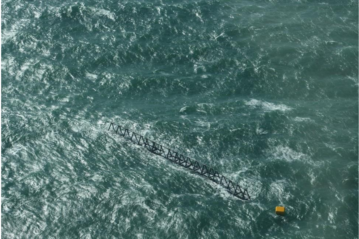
Fig. 4.3. Helicopter view of the Triton barrier during the North Atlantic storm on March 5, 2018.
