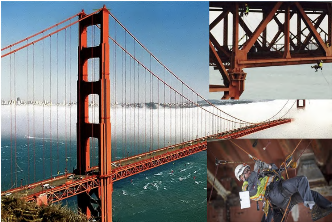
FIGURE 1.3: Current practice of steel bridge inspection: rope certified bridge engineers inspecting the Golden Gate bridge, San Francisco, California, source: NBC April 2018. Detail available here: www.nbcbayarea.com/news/local/inspections-continue-at-golden-gate-bridge_bay-area/67243/
