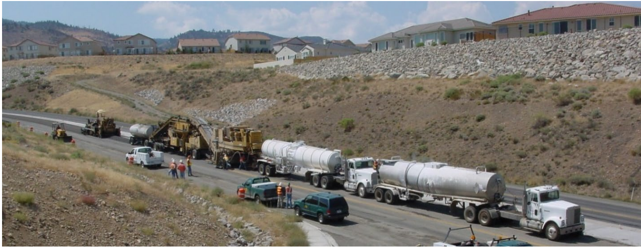
Figure 1. Picture. Cold In-place Recycling.
