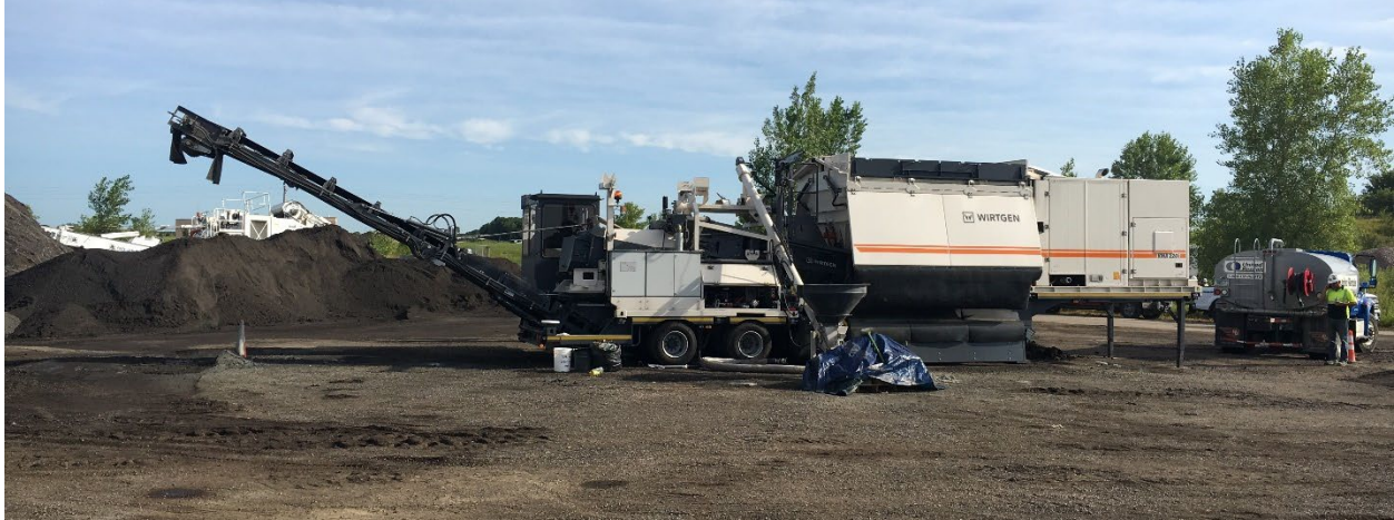
Figure 3. Picture. Cold Central Plant Recycling.
