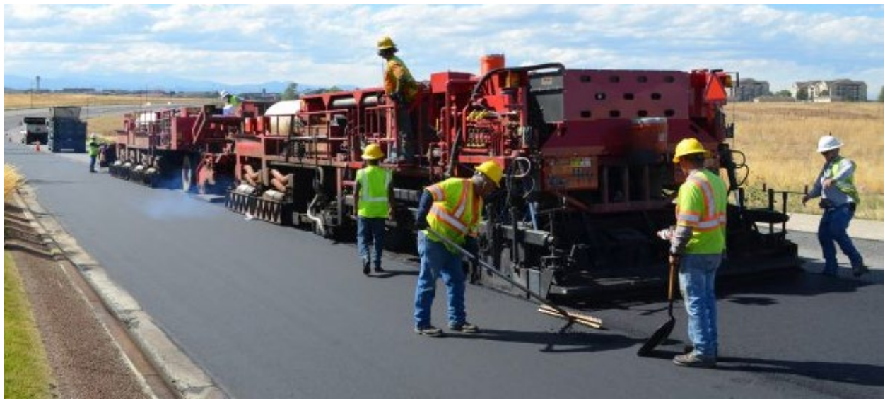
Figure 4. Picture. Hot In-Place Recycling.
