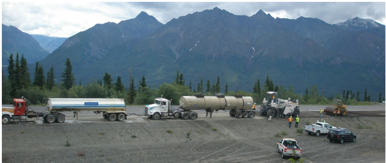
Figure 2. Picture. Full Depth Reclamation.
