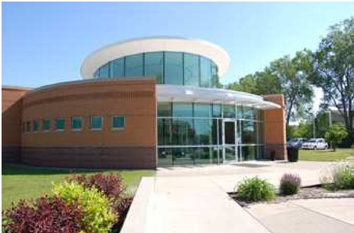
FIGURA 5.1.4 – Polk County Juvenile Detention Center, Polky County, Iowa, EUA (Fonte: POLK COUNTY IOWA, 2007).
