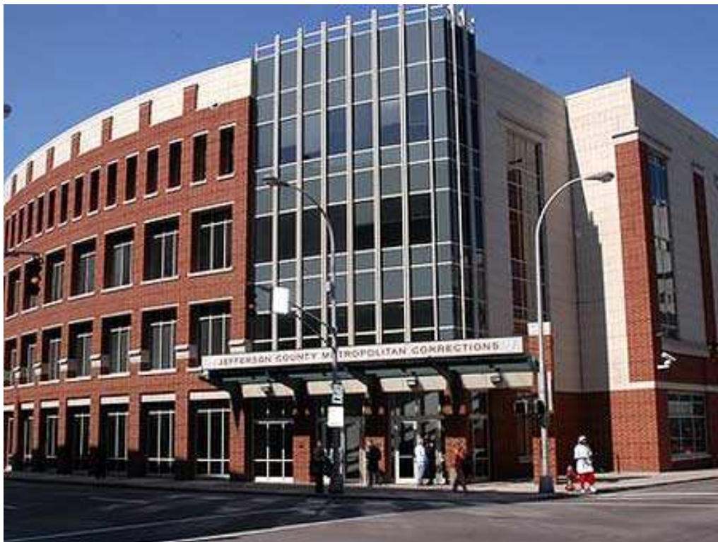
FIGURA 5.1.8 – Jefferson County Metropolitan Corrections, Louisville, Kentucky, EUA (Fonte: GOVERNO DE LOUISVILLE, 2007).
