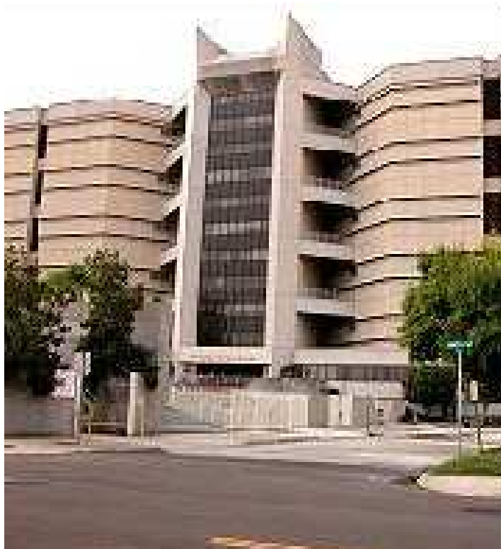
FIGURA 5.1.6 – Duval County Pre-Trial Detention Center Building, Jacksonville, Florida, EUA (Fonte: CRIME LIBRARY, 2007).
