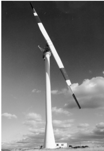
(c) Free-standing steel tubular tower of the MOD-2 [26]
