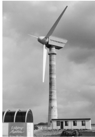
(b) Concrete tower of the Tjaereborg test turbine [26]
