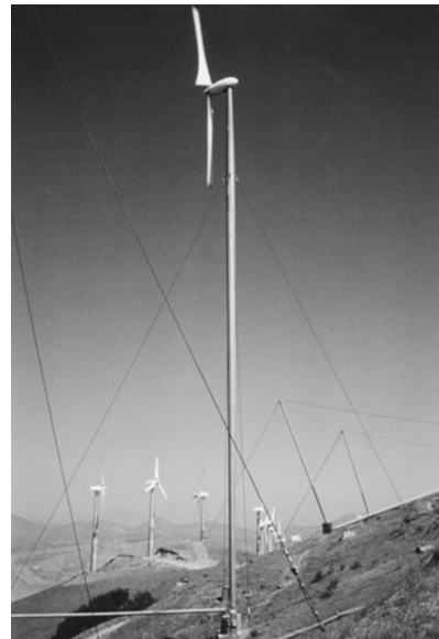
(d) Guyed steel tubular tower of a Carter turbine [26]
