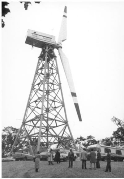
(a) MOD-1 with lattice tower [26]
