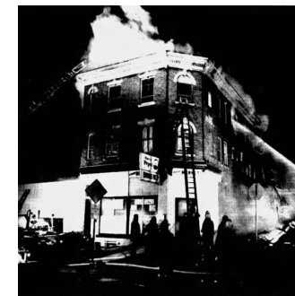
1980 fire gutted the structure, requiring extensive structural rehabilitation
